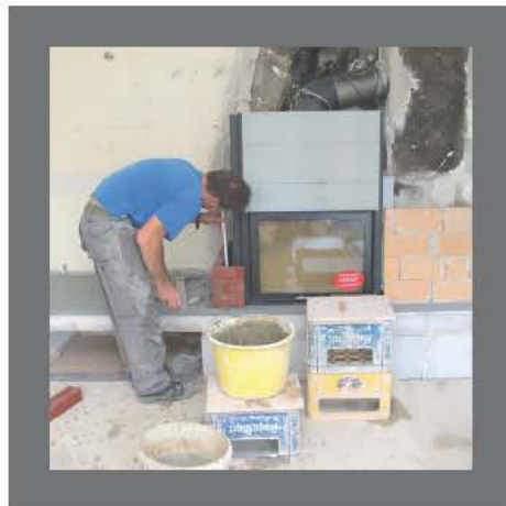
The flue gas connecting pipe has been connected up and now the fireplace insert is bricked in.
