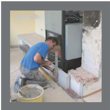
Now the stove fitter is 'setting' the heating chamber.
