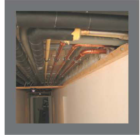
The flow and return pipes are laid in an opening in the basement ceiling and connected up to the fireplace insert.
