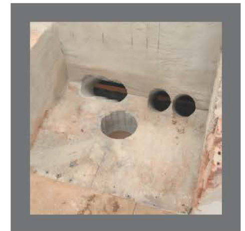
Holes drilled through the basement ceiling for the separate combustion connection and the flow and return pipes.
