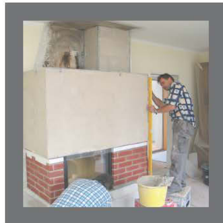
The plastered overlay is carefully skimmed and inspected.
