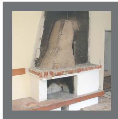
Demolition of the open fireplace and flue.
