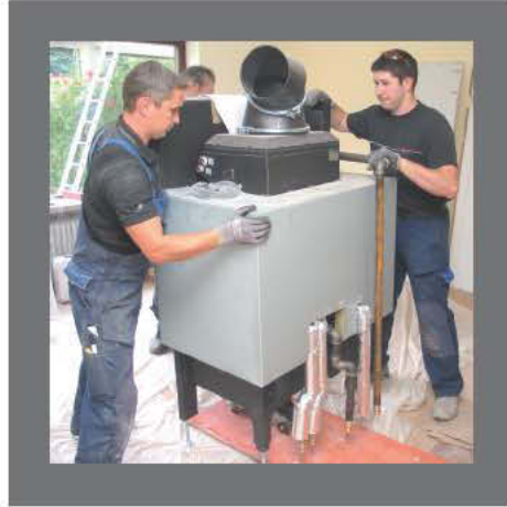
Fireplace insert pipework for the water connections and alignment of the flue gas connecting pipe outlet.
