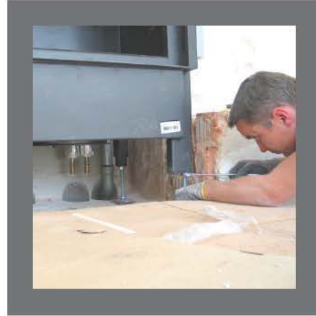
It's in its final position, the connections line up with the pre-drilled holes and the insert can be aligned.
