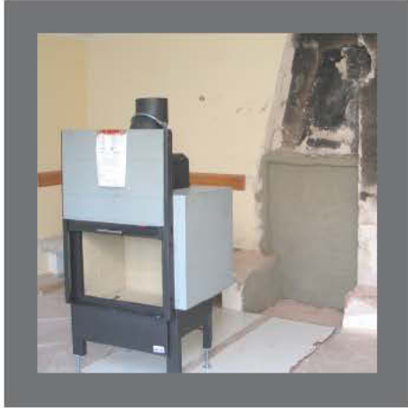
Fireplace insert awaiting installation in the living room.
