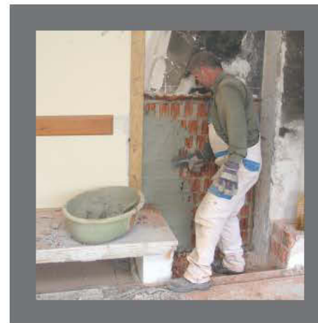
Plastering of the bare brick wall after reconstruction is completed.
